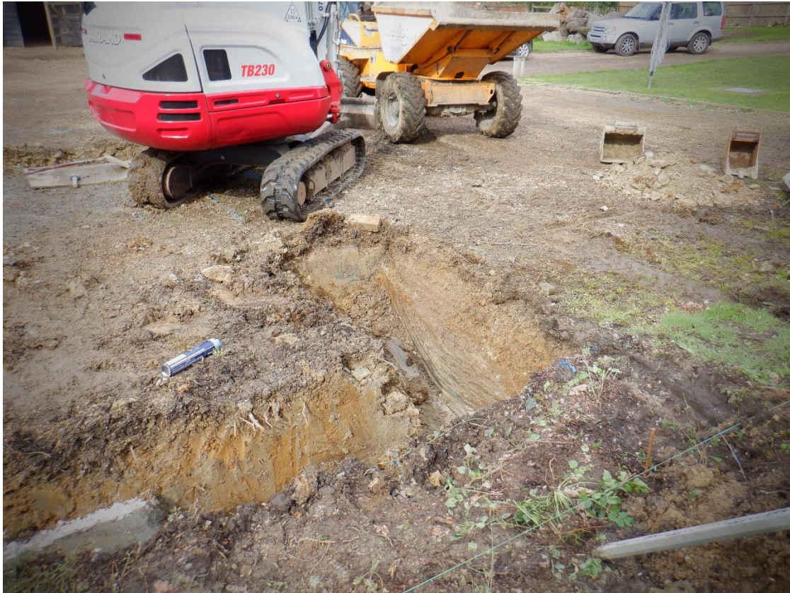
Plate 3. Day Two Foundation trenching (looking NNE)
