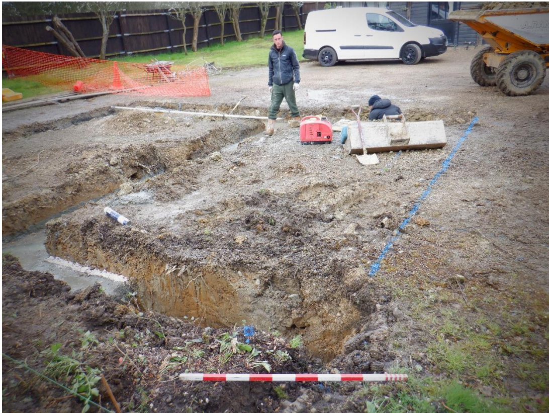
Plate 6. Day Two Foundation trenches (looking NE)
