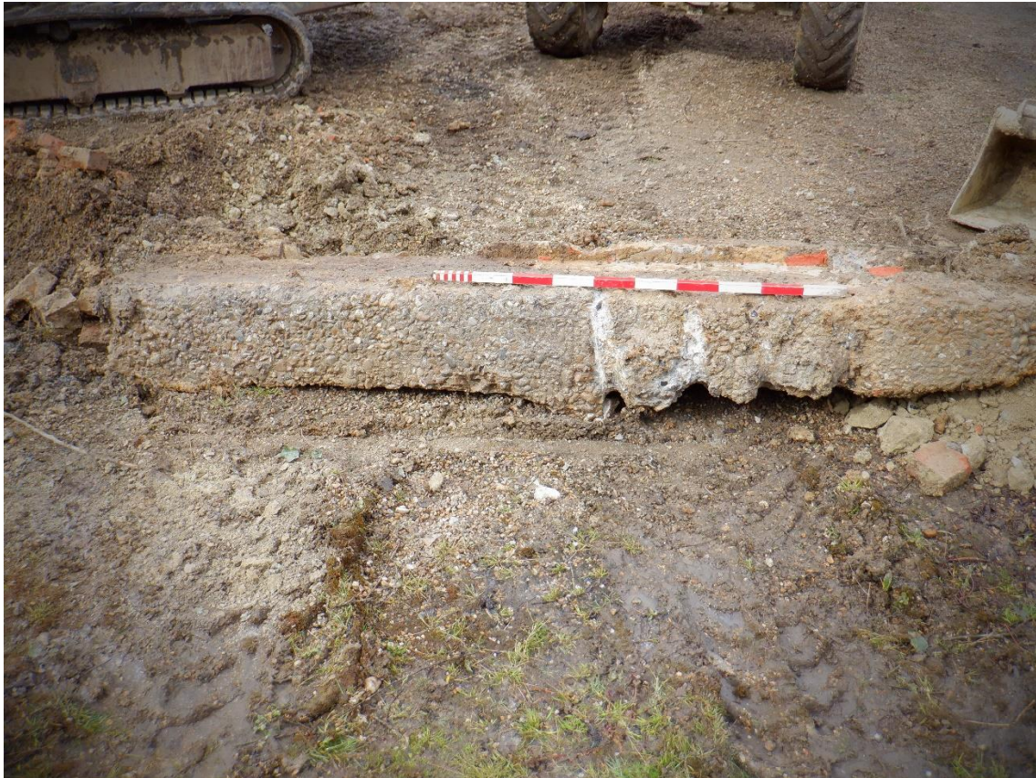
Plate 1. Removing concrete foundation footings of earlier building (looking North)
