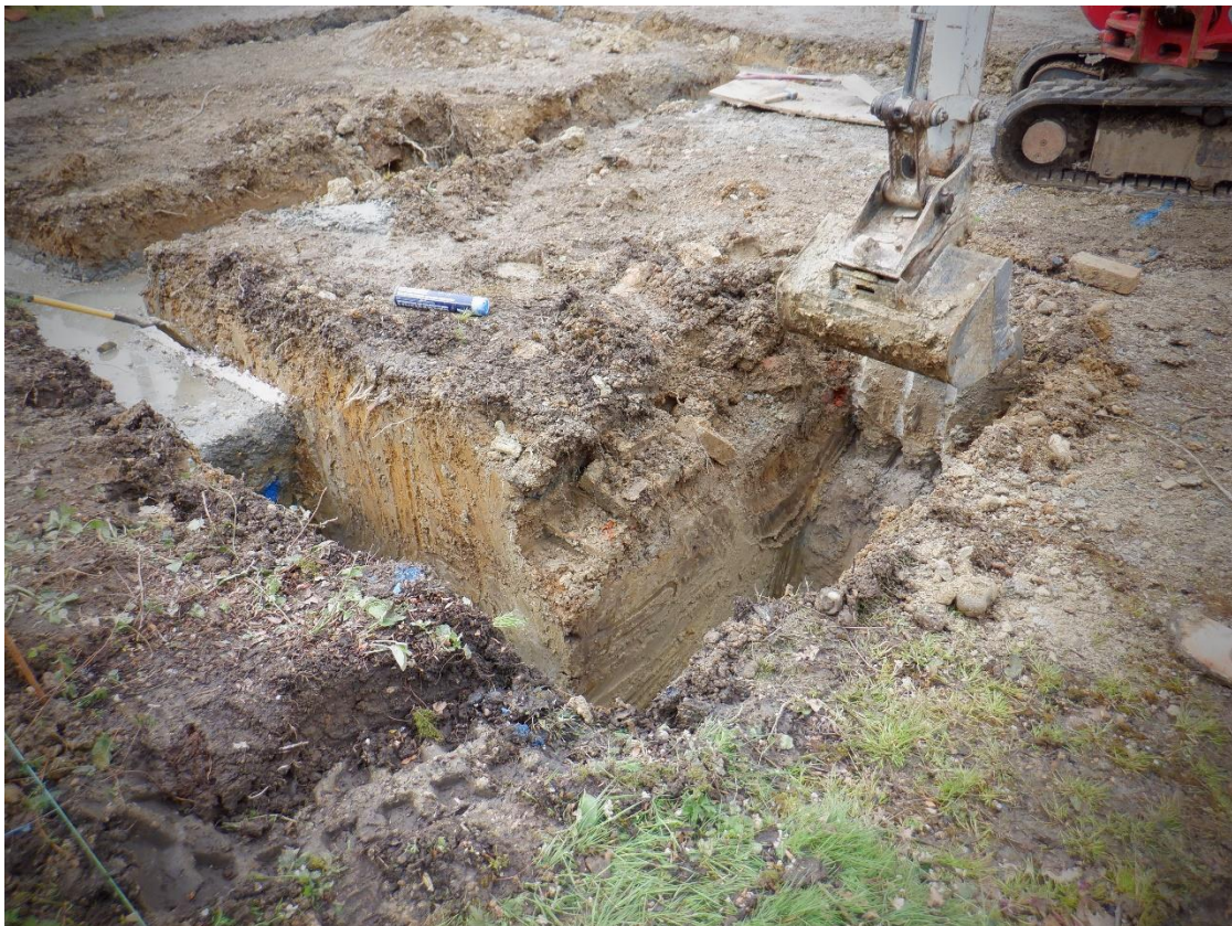
Plate 4. Day Two Foundation trenching (looking East)
